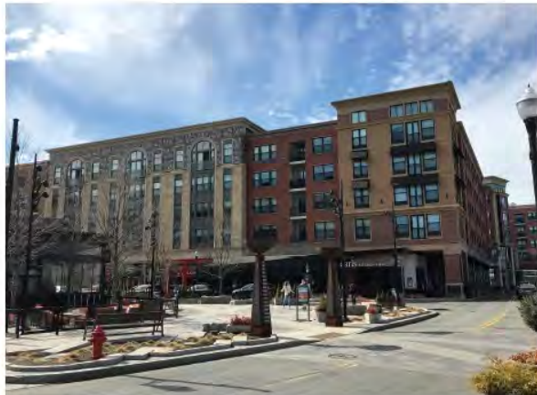
At Assembly Row in Somerville, MA, demise lines break a single large building into a collection of smaller ones.
